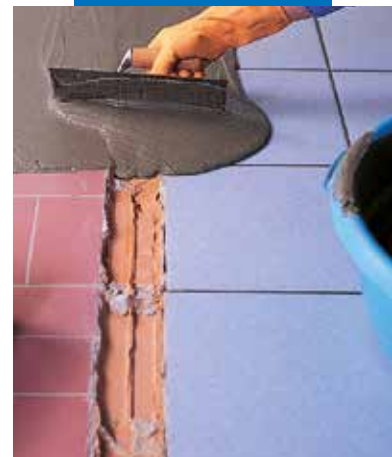
Smoothing existing flooring with Adesilex P4
