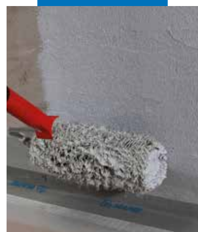
Application of Mapegum WPS with a roller
