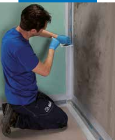
Application of Mapeband PE 120 using Mapegum WPS
