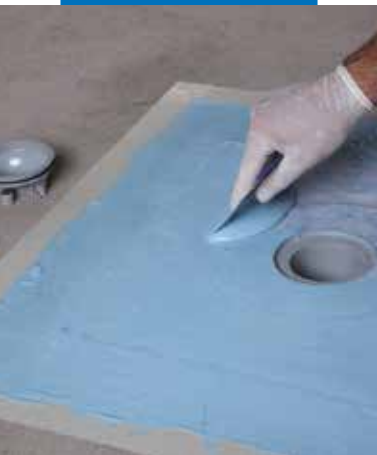
Impregnating Drain Vertical fabric with Mapelastic® AquaDefense
