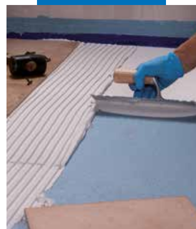
Bonding tiles on Mapelastic® AquaDefense
