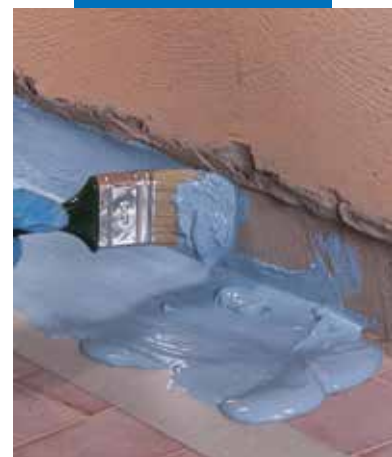
Application of Mapelastic® AquaDefense by brush between floor and wall before applying Mapeband
