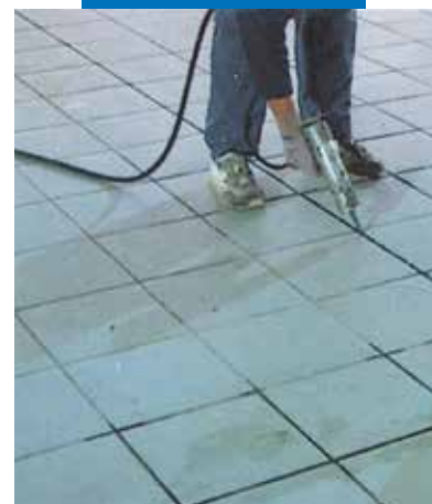
Sealing ceramic tile floor with Mapesil AC
