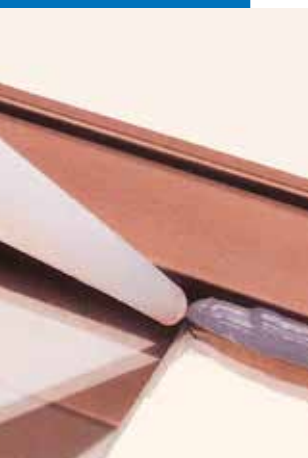
Sealing aluminium window frame with Mapesil AC
